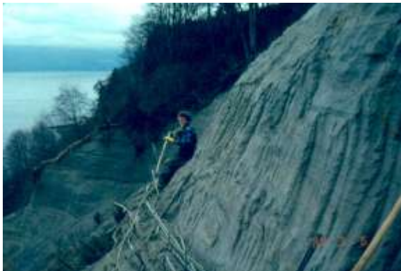
Photograph 5 & 6. This 70° sand slope below the Anthropology Museum at the University of British Columbia was treated with soil bioengineering in 1989 (left). By January 21, 2016, the slope was well on the way to becoming a forest again with Red Alder, Western Hemlock, Swordferns and Salmonberry as well as other forest species.
