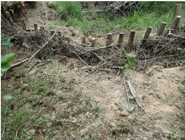
Figure 4. Sediment accumulation at FBD
