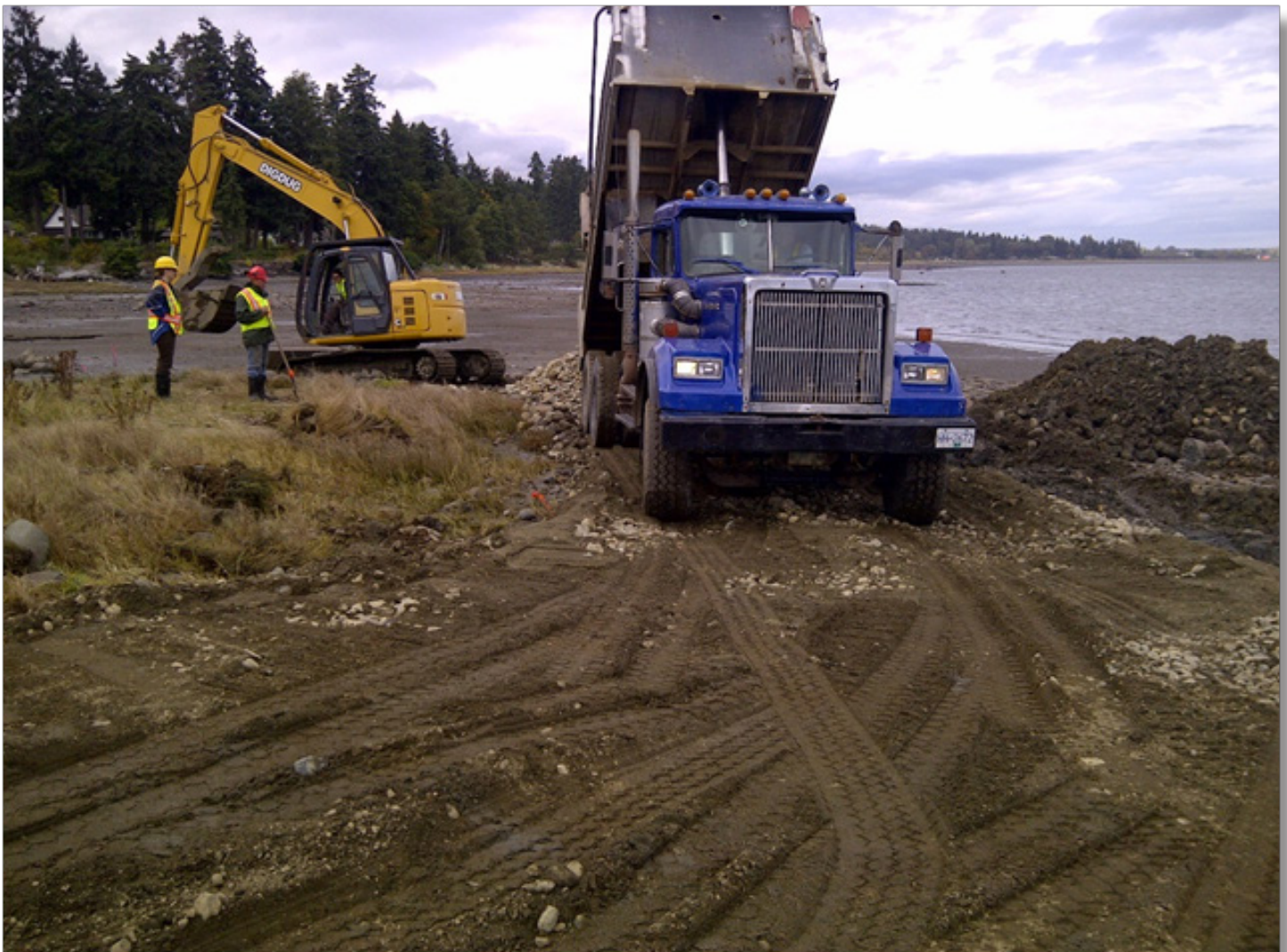
Figure 2: Construction of the berms.
