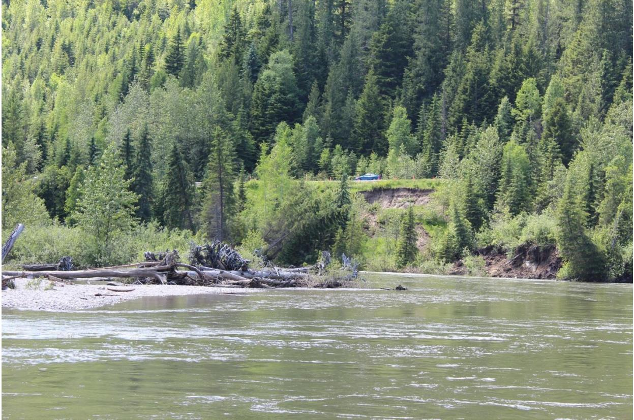
Bank stabilization was accomplished with rip rap, a permanent solution to protect Highway 5 from mass wasting. On top of the boulders, biologists placed a horizontal brush layer of willows, a bioengineering method which will continue to grow, stabilizing the soil and adding organic material to the riparian zone. Willows extending over the stream will provide cover and allochthonous energy to the aquatic environment.
