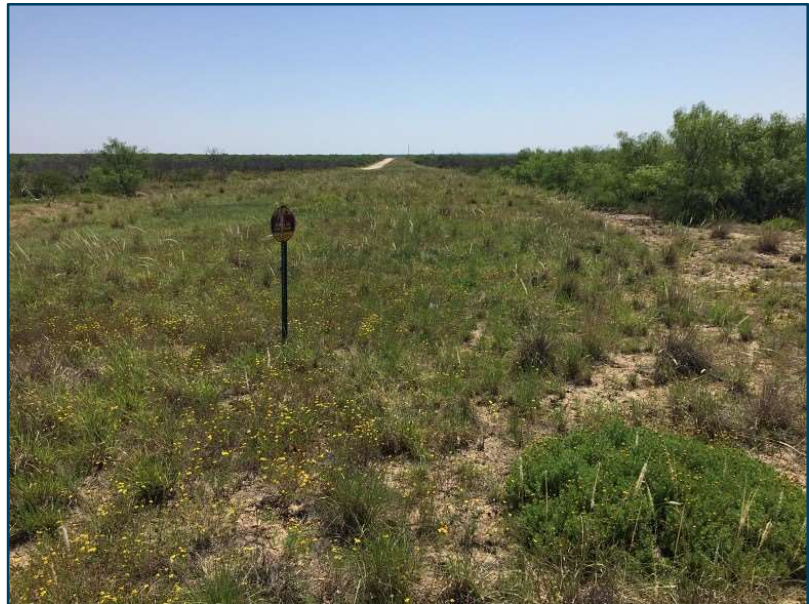
Eagle Ford Shale Pipeline – restored by private landowner and energy company. Photo credit: Forrest S. Smith
