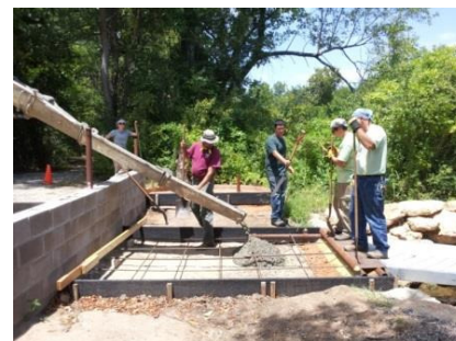
Interns and staff pour concrete for an access ramp for a floating dock.
