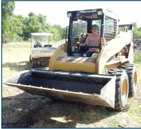
FWNCR Intern preparing to load soil into the skid steer bucket.
