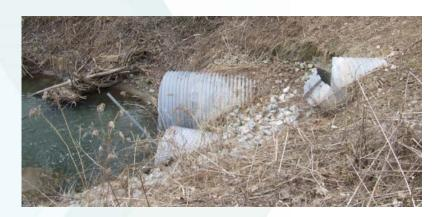
Culverts were rusting out, and erosion was present both upstream and downstream of culvert
