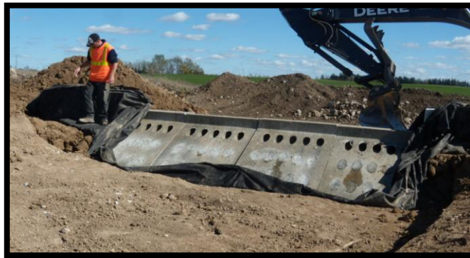
Figure 4: Construction of Berm 2 on the Eadie Farm
