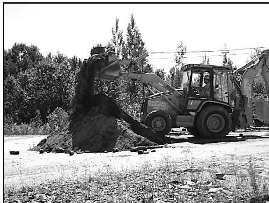
Figure 2: Backhoe mixing finely crushed mine rock and woody residuals on site at Barrick (Hemlo, ON).
