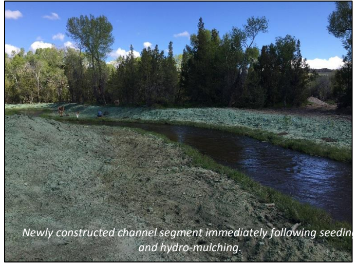
Construction of narrower channel adjacent to infested segment of Jefferson Slough.
