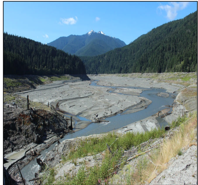
Figure 1. View of the former Lake Mills reservoir (July 11, 2013). There is still 50 ft of dam left, so the river in its current location is 40-50 ft above the original valley bottom.
