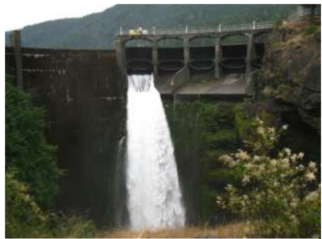
Glines Canyon Dam (A. Clausen).
