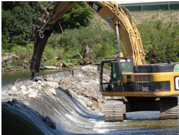
Removal of the Fifth Avenue dam in August 2012
