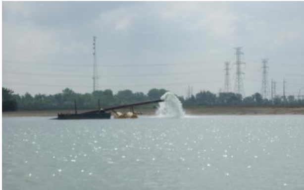
Hydraulic dredging of lake bottom to create sand islands
